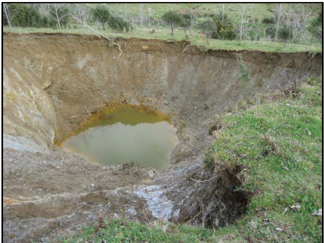
Figure 4-3 Debris filled sinkhole 26 July 2013
