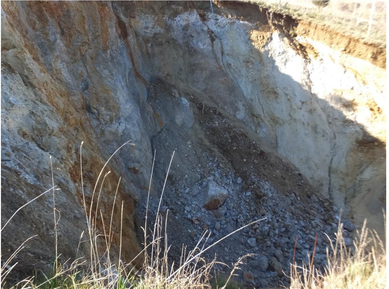
Photo 2. View of the sink-hole crater showing a fan of slope failure debris from the eastern side resting on the crater floor.
