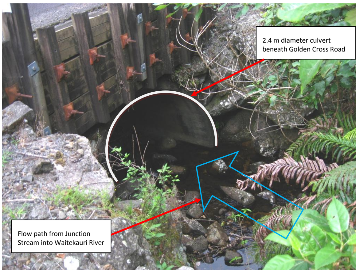
Photograph 4. 2.4 m diameter culvert beneath Golden Cross Road through which the Junction Stream discharges into the Waitekauri River
