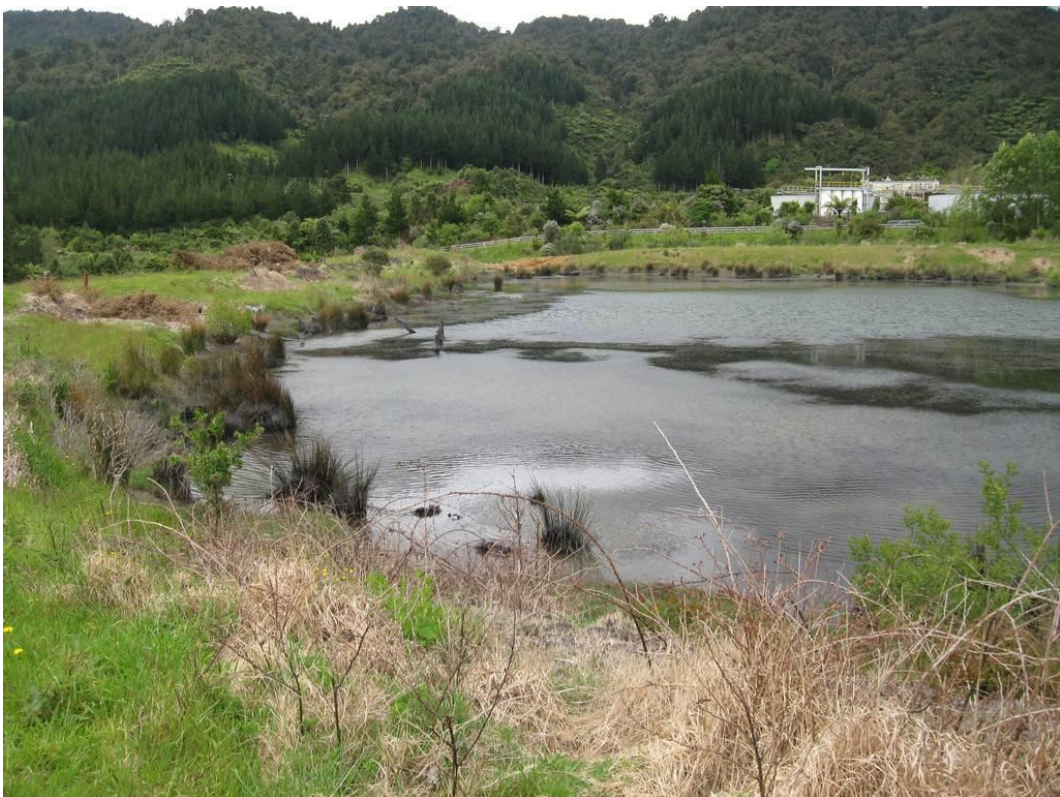
Photograph 7. Looking along USD embankment (left) towards spillway
