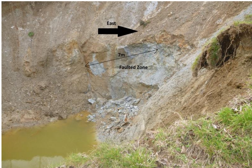
Photograph 4: View of the fault zone
