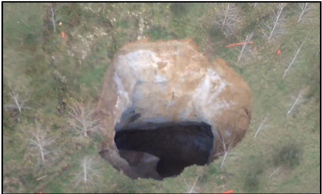
Figure 4-2 View from Helicopter into sinkhole 14 June 2013 (taken from Tonkin & Taylor video footage)
