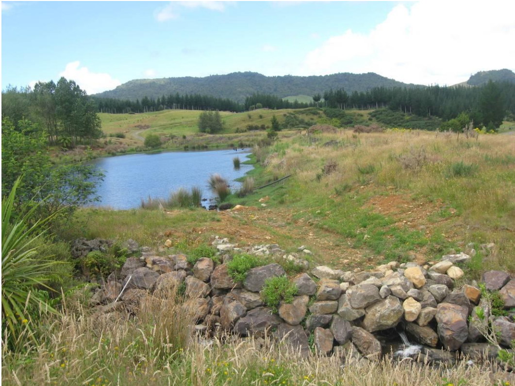
Photograph 6. Lowered USD overland spillway (pipe discharge approximately 0.5 m below spillway level)
