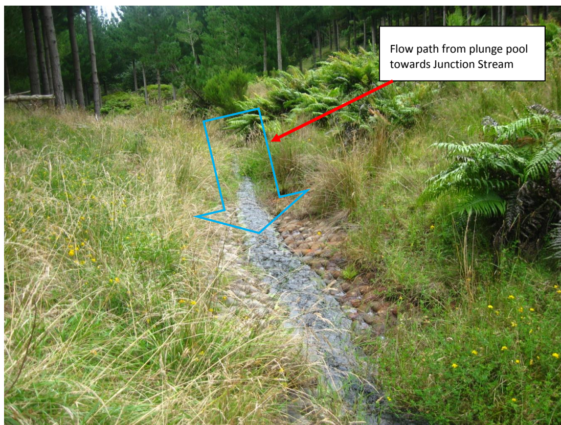
Photograph 3. Looking upstream along concrete-lined channel towards plunge pool
