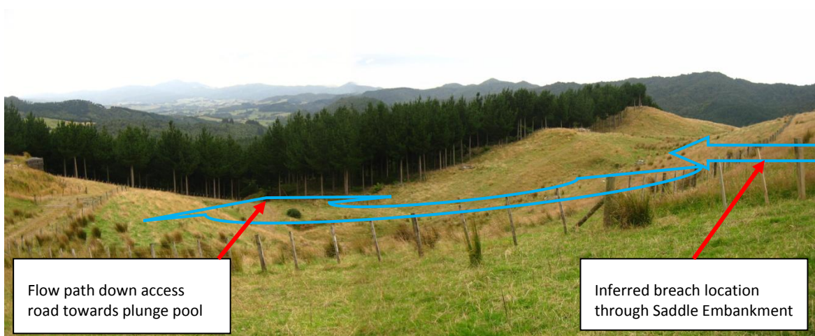
Photograph 1. Inferred flow path of possible dam breach release
