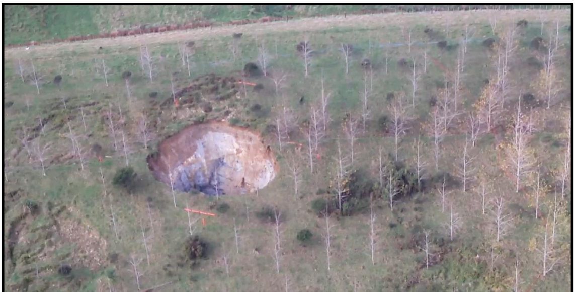
Figure 4-1 Aerial view of sinkhole 14 June 2013
