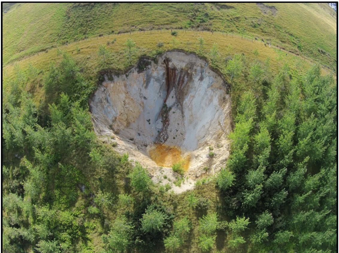
Figure 4-8 June 2015 sinkhole images from aerial survey drone
